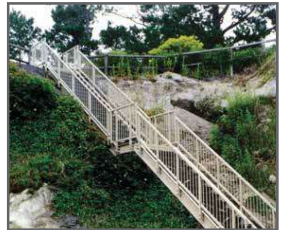
This all FRP stairway is located at a private residence in the Pebble Beach community in California. The stairway leads from the front yard of the home to the private beach below.
