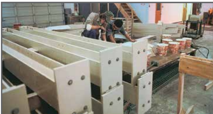
Fabricated Dynaform columns ready for shipment.
