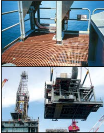
Tension Leg Platform
