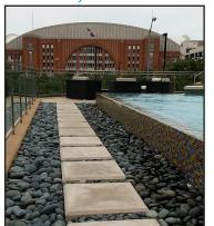
Fibergrate molded grating and quad head pedestal legs were used over this pool's drainage trench. It was then covered with a synthetic mesh, as an added filter for trash and debris, before being covered with river stones and walking pavers resulting in a secure walkway and drainage around the exterior of the pool.
