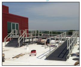
Some sections of the of the platform were fabricated on the ground before being lifted to the rooftop.
