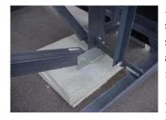
All hardware behind antennas is standard 316SS or galvanized steel. Any hardware in front of antennas where RF transparency is a concern is 100% fiberglass.
